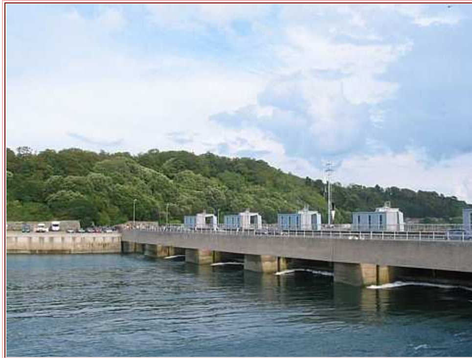
Photo 4 Tidal power barrage at the estuary of the Rance River, France (From EnergyBC, Ref. 6)
