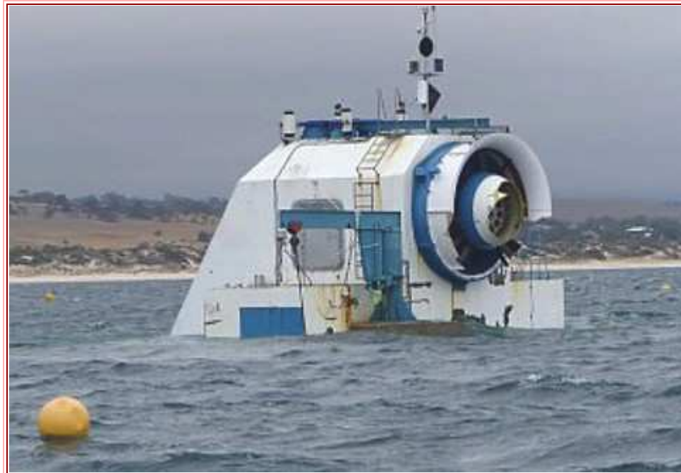
Photo 3 The Oceanlinx Wave Generator on the Ocean floor at Carrickalinga
