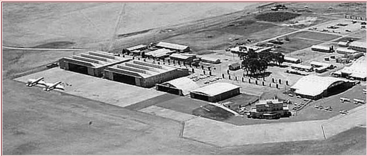
Photo 18 - Department of Aircraft Production (DAP) 1965. The DAP hangers Hangars are the two large ones on the left. (Goodall Photos - Ref. 8)
