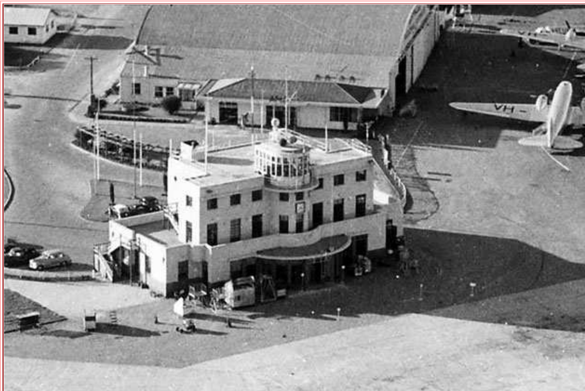
Photo 8 - Control Tower Parafield 1948 (Aerial Photos - Ref. 5)
