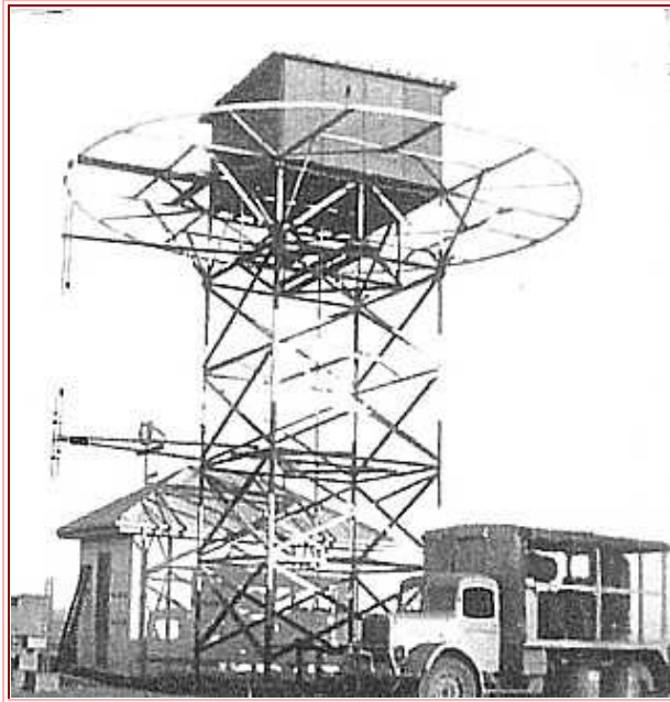
Visual Aural Range (VAR) in 1950 at Leigh Creek & Austin truck loaded with 25kVA power plant (Photo John Ward, ref 6)
