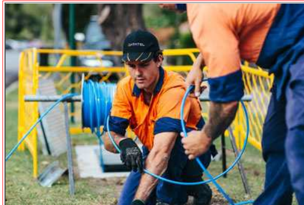
NBN Installing Fibre Optic Cable
