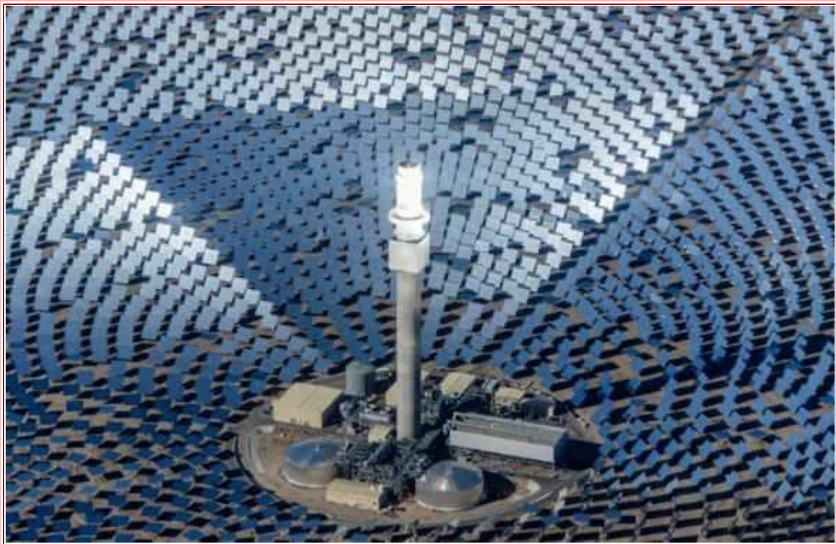
Solar towers and storage Crescent Dunes in Nevada
