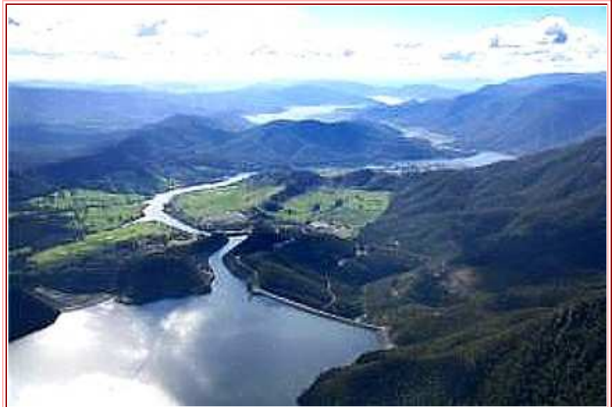
Talbingo Reservoir with its Tumut 3 Power Station Dam and Jounama Pondage in the background
