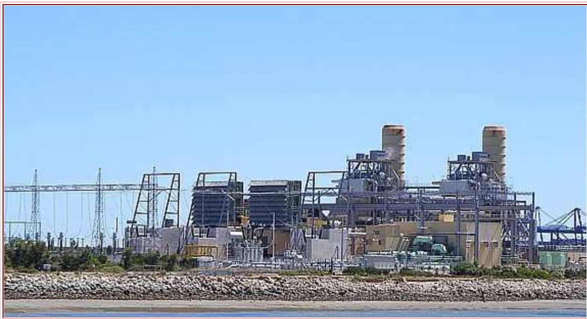
Pelican Point Power Station
