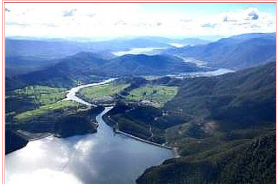
Talbingo Reservoir with its Tumut 3 Power Station Dam and Jounama Pondage in the background
