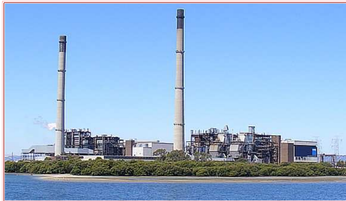
Torrens Island Power Station
