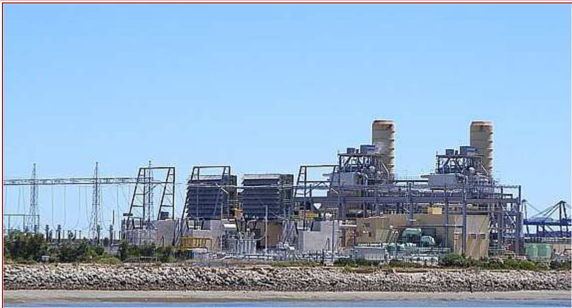
Pelican Point Power Station
