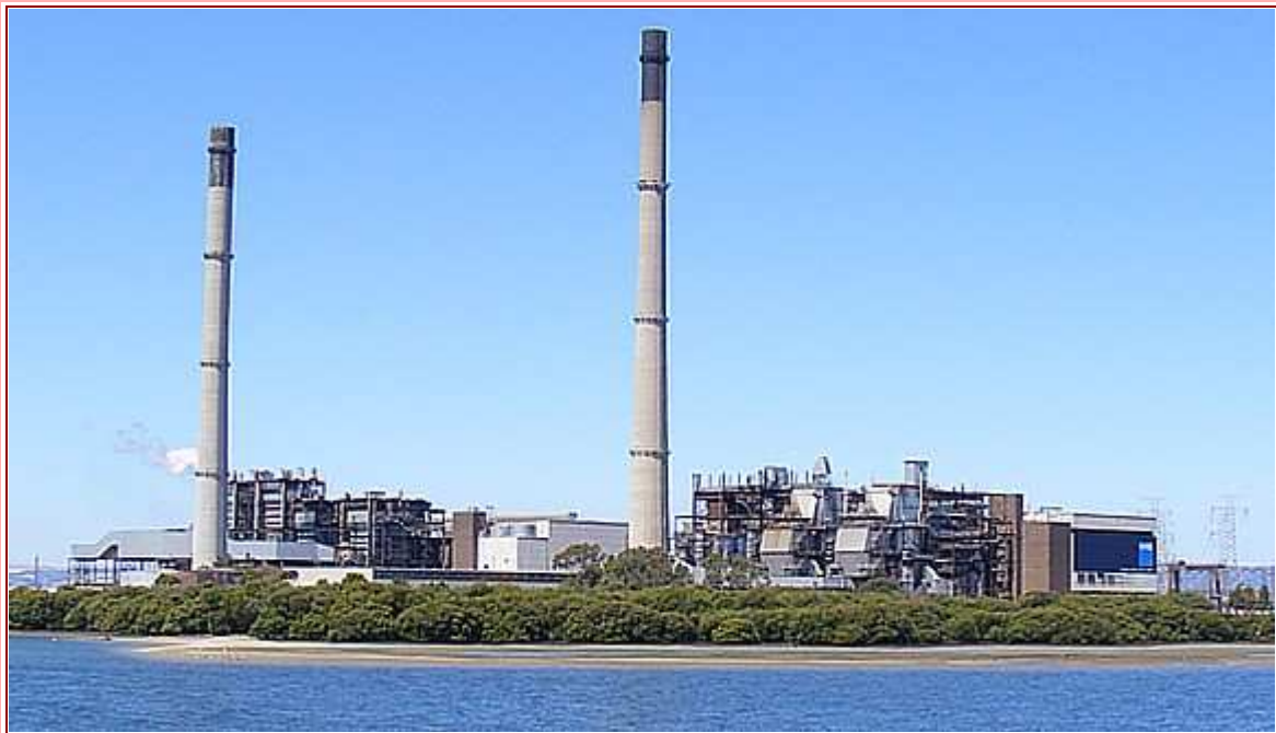
Torrens Island Power Station
