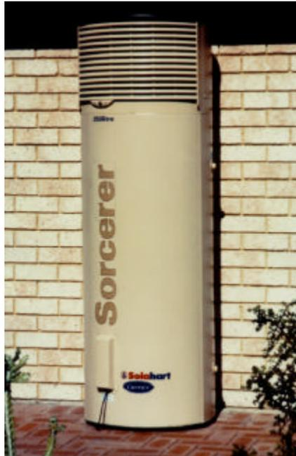
Integrated air-source heat pump water heater.
