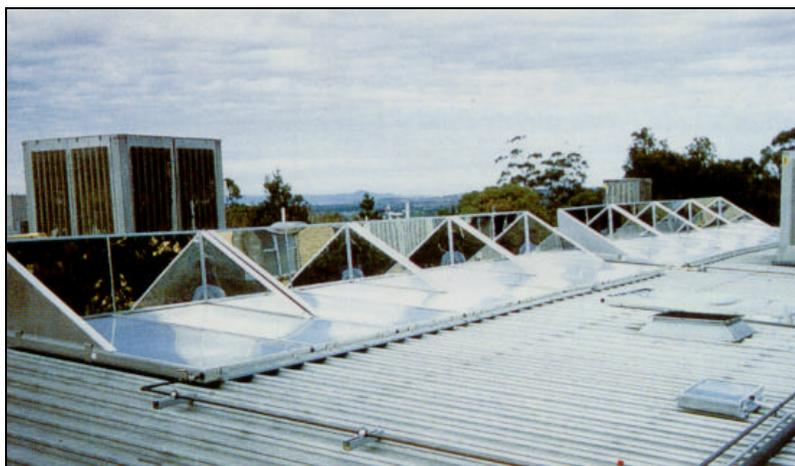
Mirror booster solar collectors on a low slope roof.
